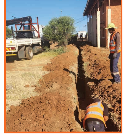
Trench preparations ; Supply and installation of 210m 11kV ; 35mm2;3C XLPE Cable in Goodhope
