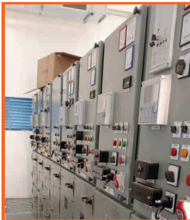
Installation of 3.3kv Switchgear in New 11kv-3.3kv Substation at Mmamashia Water Treatment Plant
