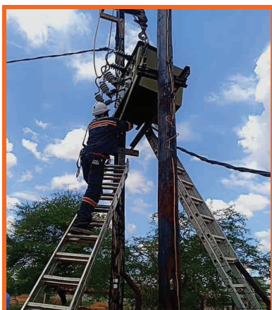
Bpc works 11KV 50KVA ;3PH Pole Mounted Transformers- Pole Replacements in Mochudi
