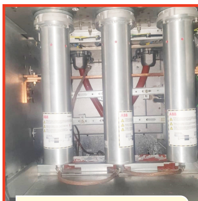
11KV PANEL LIGHTING ARRESTERS, BOTTOM ENTRY
