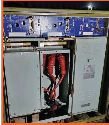
Supply and install 11kV; 35mmx3core XLPE Cable Termination in 11KV ; K3 Minisub at Goodhope Council
