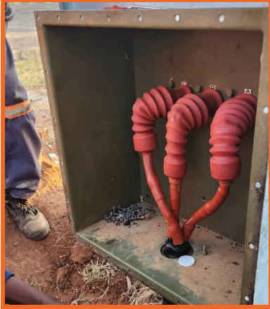
Supply and Install 11kV; 35mmx3core XLPE Cable Termination in RMU at Goodhope Council Offices
