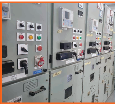
Installation of 11kv Switchgear in new Substation for the New Mmamashia Water Treatment Plant
