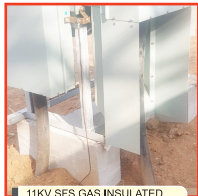
11KV SFS GAS INSULATED RMU INSTALLED
