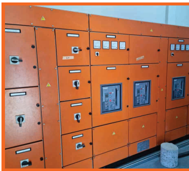
Installation of New 400V LV Board in New Substation at Mmamashia Water Treatment Plant
