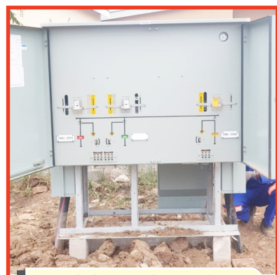
NEW SF6 RMU INSTALLATION COMMISSIONING IN PROGRESS
