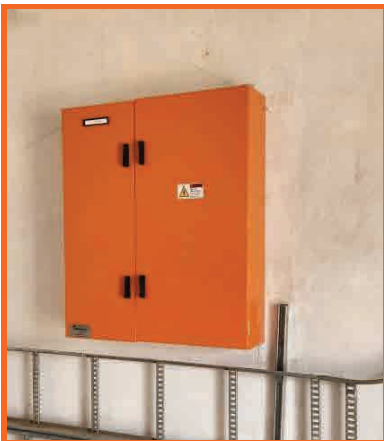
Installation of LV Distribution Boards in Inlet Tower at Mmamashia Water Treatment Plant
