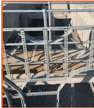
Cable Racking between Filters at Mmamashia Water Treatment Plant
