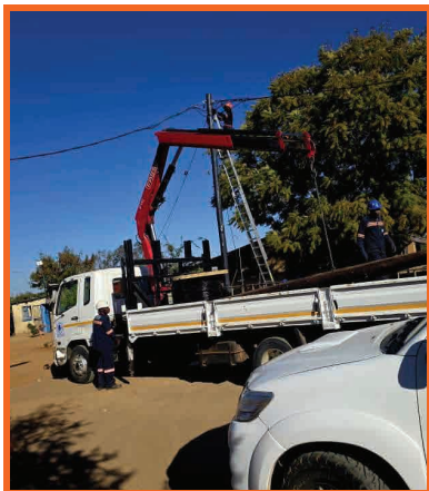
Bpc works 11KV 50KVA ;3PH Pole Mounted Transformers- Pole Replacements in Mochudi
