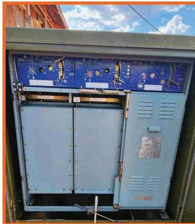
Maintenance and Servicing 11kV ; 315kV ; 3Ph ; K3 Minisub at Goodhope Council Offices
