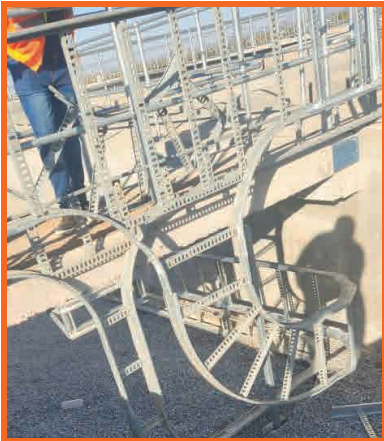
Cable Racking at Filter Area in the Mmamashia Water Treatment Plant Works-
